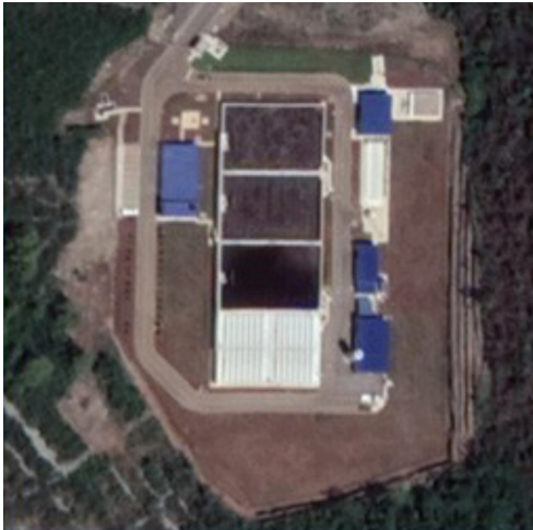
Picture - WWTP Kotor-Tivat (SBR units)
